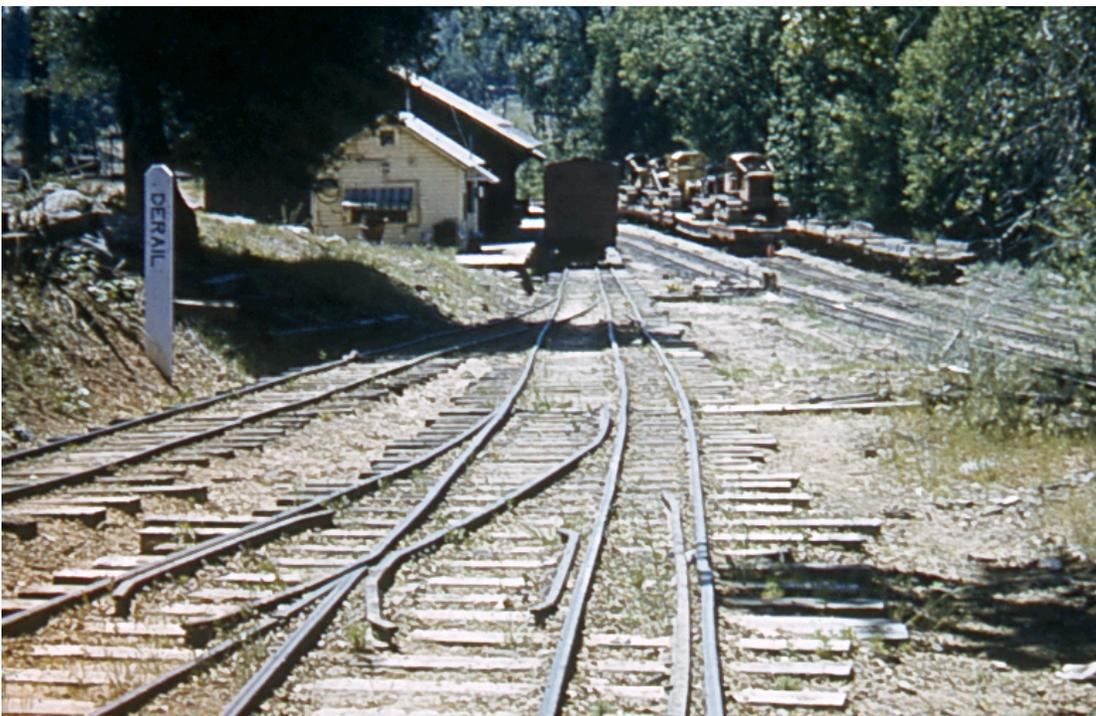
This is looking down from the wye. First track on the left is the third leg of the narrow gauge wye. Second track on left is a siding. White building on left is Dispatcher's Shack. A reefer is beside the woods warehouse for loading. A work train with 4 tractors on 4 equipment flats is on the main line and two flat cars are on the siding next to it.
