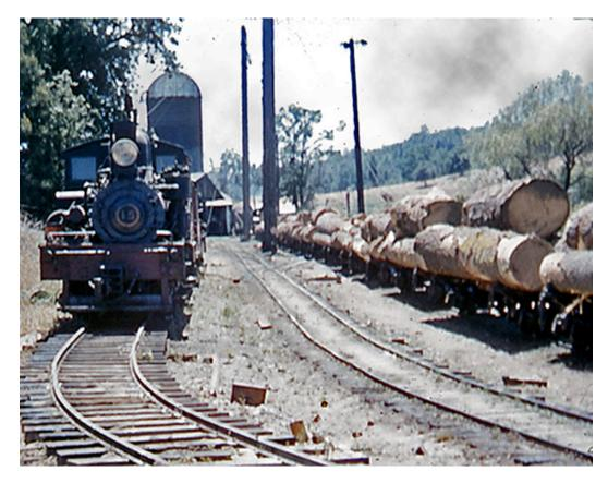
We got this close to the to the dump area before turning around to see if another train was coming. Shay no. 9 is about to be uncoupled from the log cars which are lined up along the brow log. Shay no. 15 is in the RIP or dead line at the left. Please proceed to Part Two, Section 2B, for more photos & story.
