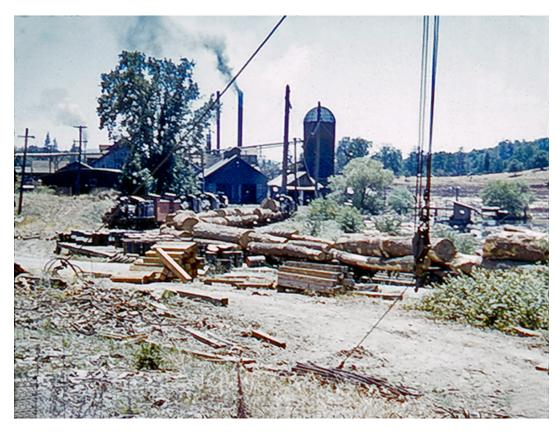
We then left the deck in front of the Dispatcher's shack and went around behind the woods warehouse to watch the train head for the log dump. The train was nearing the brow log. The RIP (repair in place, usually) track was at the left. I also heard it called the "dead line". The mill, with the engine house in front, the speeder and straddle carrier repair shed, and the slash burner were in the distance. At right
