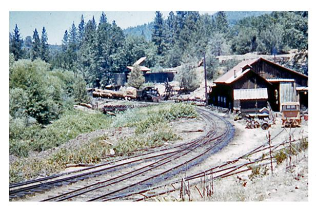
As the train first appeared, many details of the area could be seen. Gas switcher no. 1 is at the right; the platform and high pressure water nozzle for washing empty log cars was at its left. Behind that was the blacksmith's charcoal storage shed.
