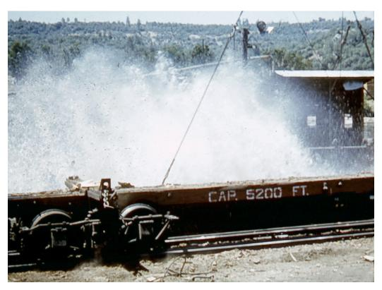
This was my first photo of the dumping at the log pond. In the background was the winch house, with two winches that controlled the two cables that were used. The winches were steam powered; the steam was piped to the winch house from the mill's main boiler. using a very long pipe that was wrapped in asbestos insulation. This pipe can be seen here entering the winch house.
