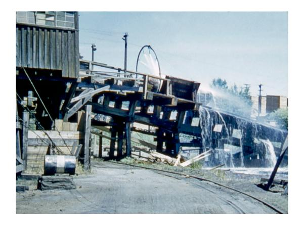
Before leaving the pond area, I quickly went around the mill and photographed the tail track and the jack chain that brought logs from the pond into the mill. Logs were washed to remove loose debris so the band saws would not throw the debris around where men were working.
